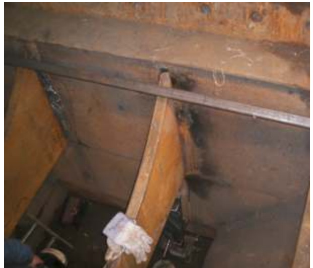
After the repair
