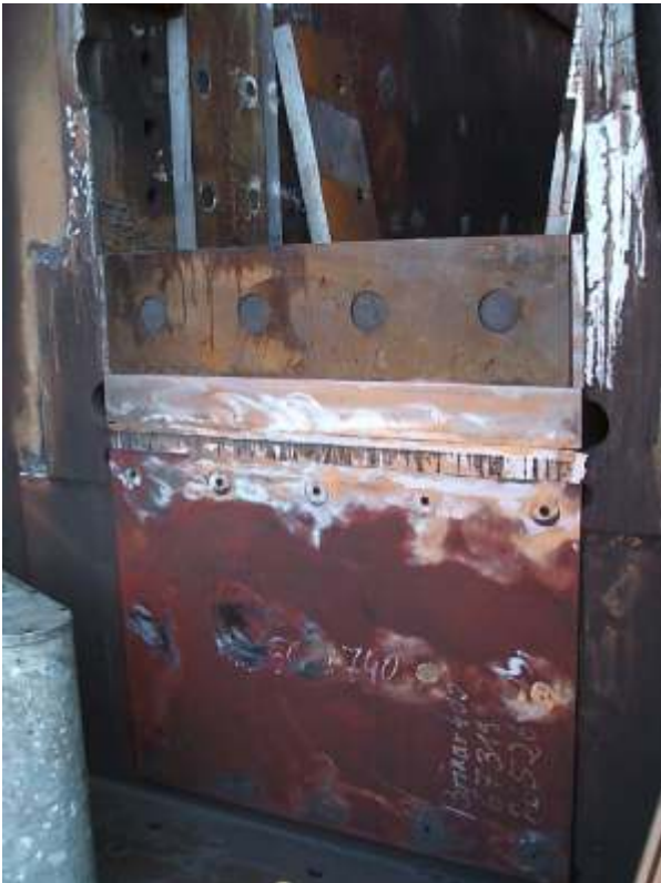
Frame after repair
