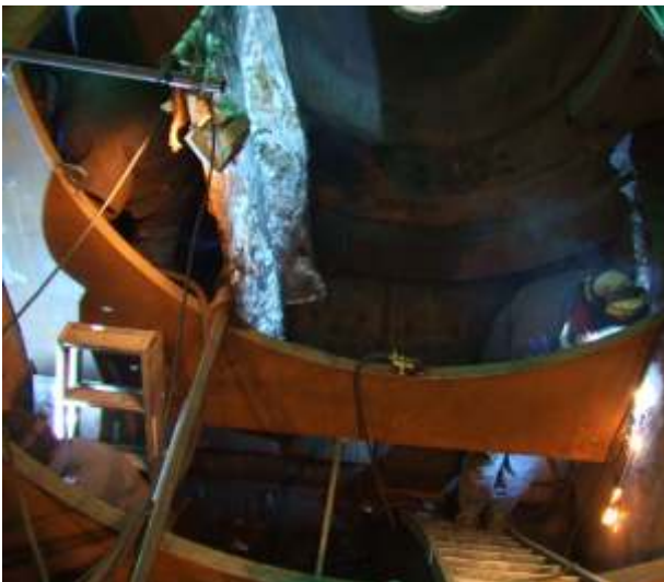
During the repair
