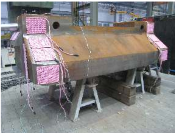
Fix the heating mats
