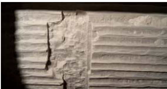
Roller Body cracking and flaking
