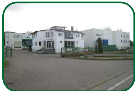
Expansion of the manufacturing plant Seiferstraße 16
